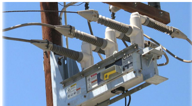
Figure 21: Example – Distribution line recloser.
