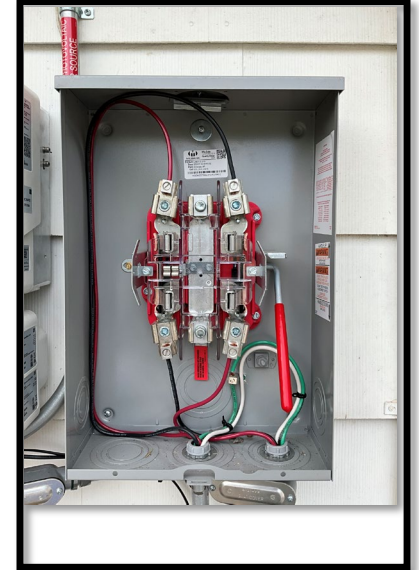
Production Meter Wired Backwards
