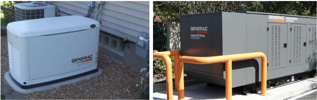
Figure 46: Example Residential and Commercial/Industrial Natural Gas Generator Sets
