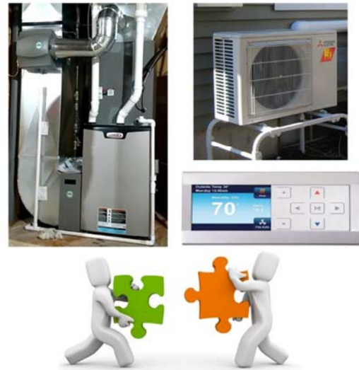
Figure 18: Natural Gas and Electric Hybrid Heating Systems
