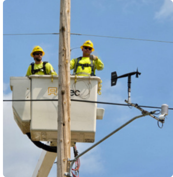
Linemen installing a weather station outside of Rapid City, South Dakota
