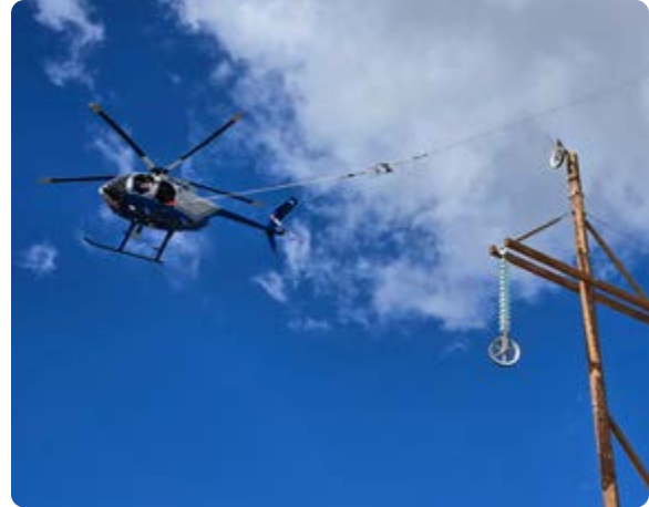
An expertly piloted helicopter installing transmission lines
